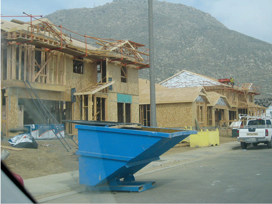
These homes are in the process of having the wood sheeting installed. That is Blue Mountain in the background.
