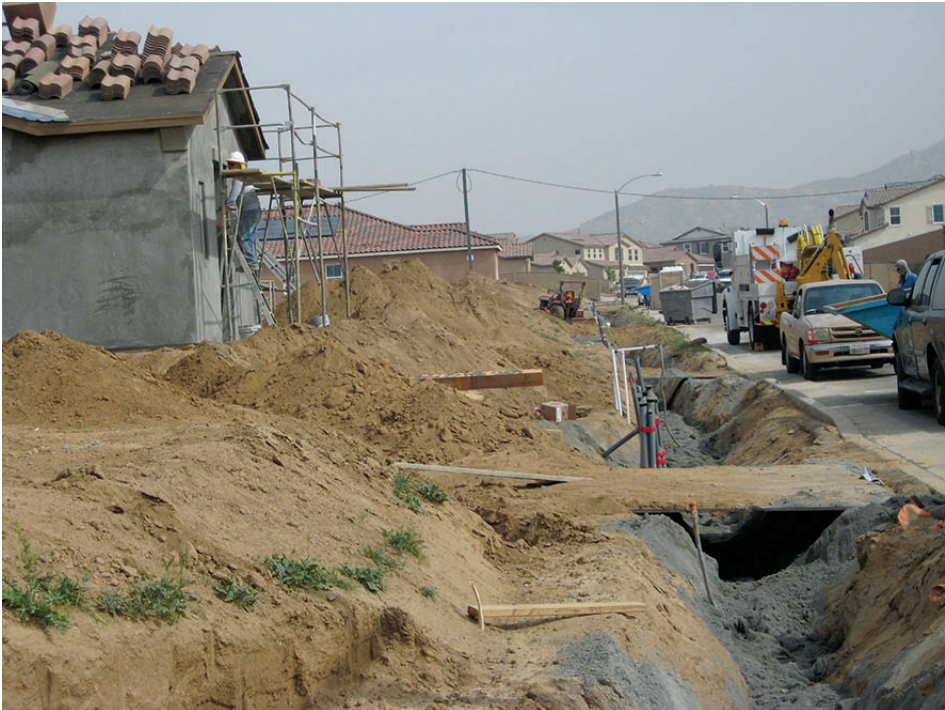
This house is receiving the stucco and the roofing is ready to be installed.
