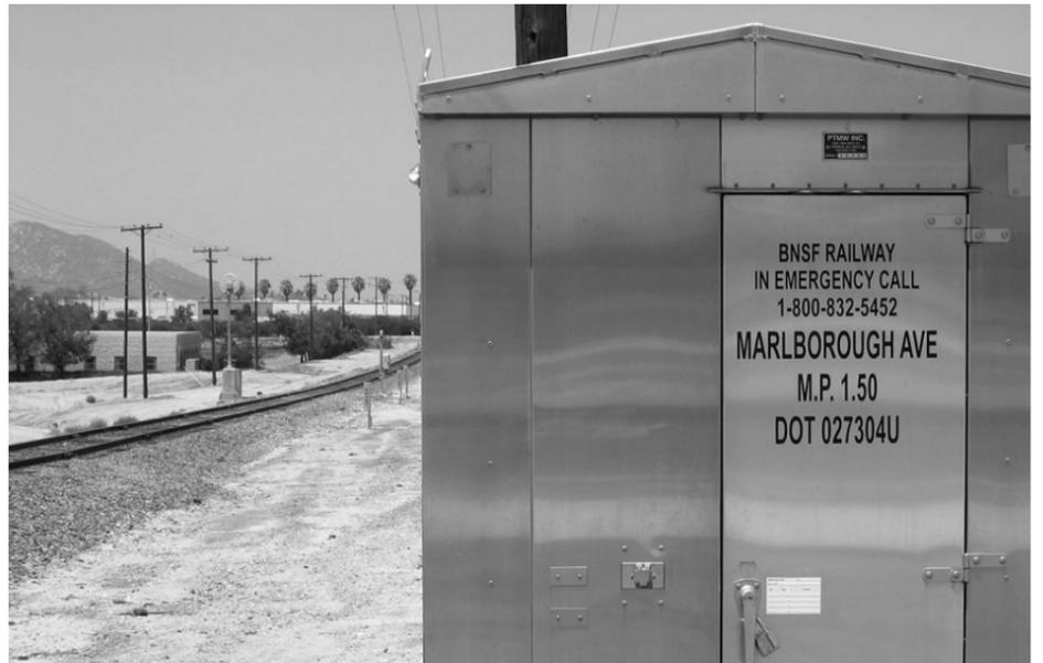
This electrical box is the only signal system on the 38 mile Perris Valley Line track. It is used to stop other trains on the Riverside Line track, owned by the UPRR, that crosses the Perris Valley Line track at Marlborough Avenue. It is not a CTC signal governed by the train dispatcher. When it is red, trains on either railroad know there is another train crossing ahead of them. It is similar to a traffic light at an intersection.
