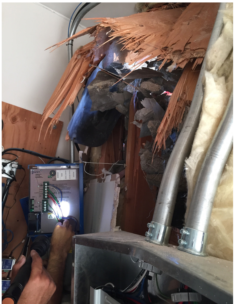
The impact damaged the electrical panel in Chevron's storage room.
