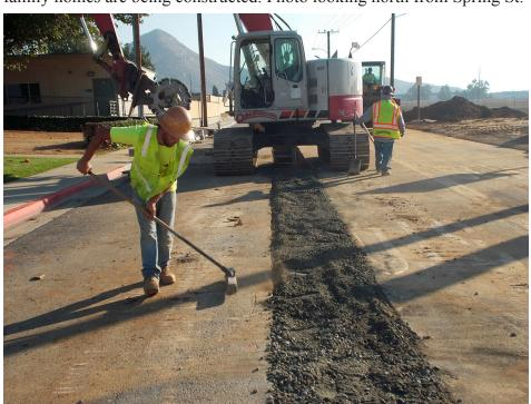
This view shows workmen by the school on Garfield covering up the new sewer line that will tap into the existing sewer line along Center Street.
