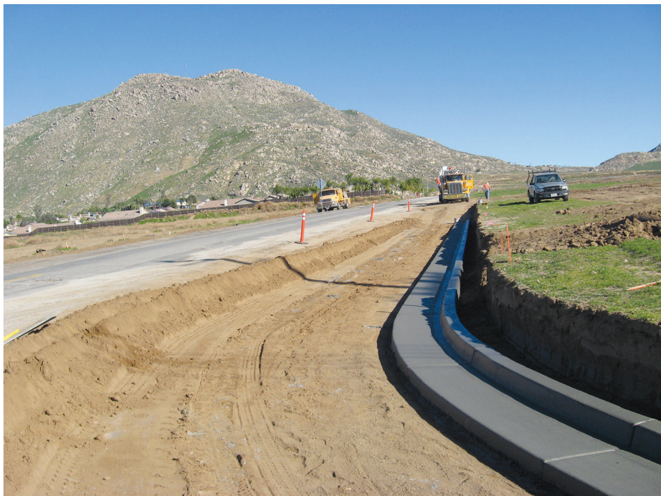
New curb and gutter is part of the Spring Mountain Ranch improvements. This photo shows Center Street east of Mt. Vernon Avenue.
