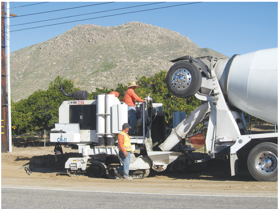
This machine makes the curb and gutter. This was taken on Jan. 6, 2015 next to one of Highgrove's last orange groves north of Mt. Vernon Ave.
