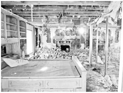
The upstairs bedroom had estensive damage to the ceiling, roof, and trusses and there probably was water damage to both the top and bottom levels. This is the view of the upstairs bedroom. The bricks from the wall had to be removed to allow firemen access to the wall that was smouldering.
