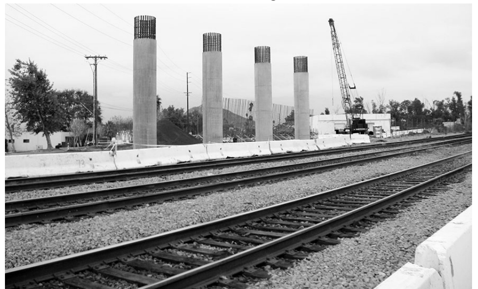
Iowa Avenue Overpass
