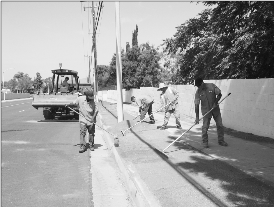
County Transportation workers recently installed decomposed granite between the curb and sidewalk along Center St. in Highgrove. It really looks nice!
