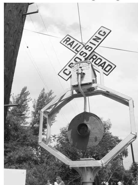
This early railroad crossing warning system is referred to as a "Wig-Wag". The round part in the middle swings back and forth to warn motorists of an approaching train. (Cont. on P. 5)
