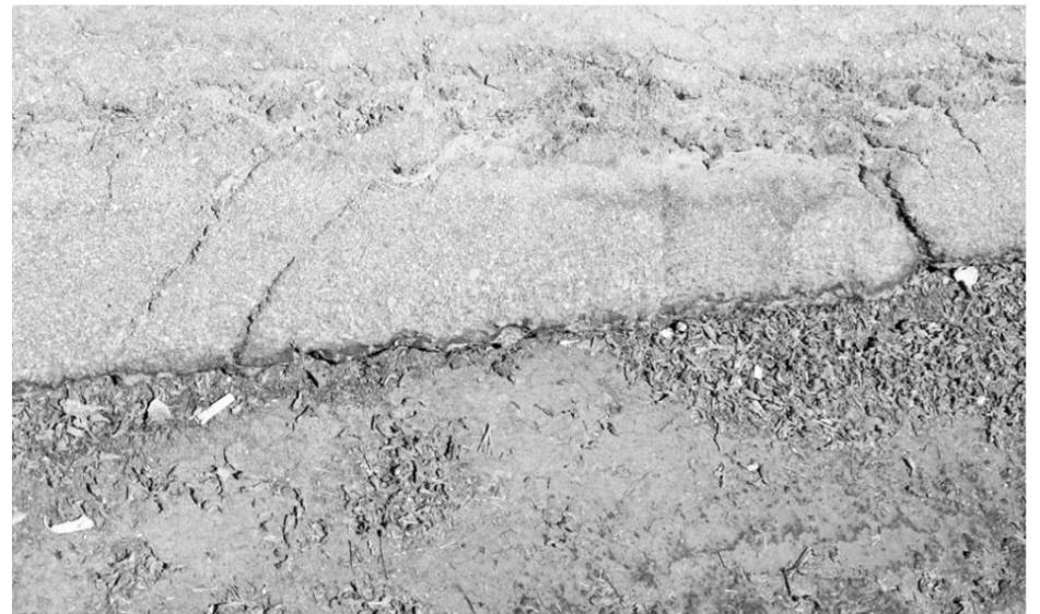
When new construction begins, the curb and gutters should be made of concrete. The cheaper asphalt curbs get soft in hot weather and crush when they are ran over. Concrete curbs last much longer!
