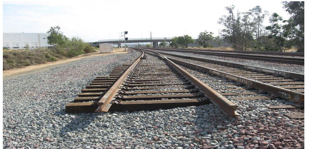
The new switch is in place from the BNSF RR that will go to the Perris Valley Line railroad track. The Iowa Ave. overpass is shown in the distance.
