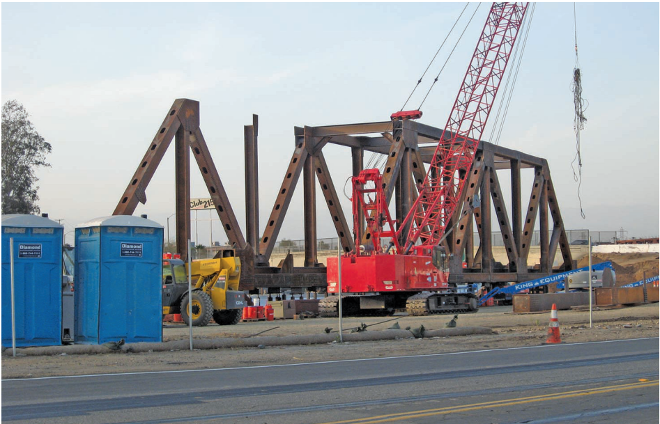
The 5th section of the railroad bridge is shown during construction that is underway directly across from the Yum Yum Restaurant in Colton. There are already 4 new bridges like this over the freeway but a 5th and 6th section will enable a 3rd main line over the I-215 instead of the present two.
