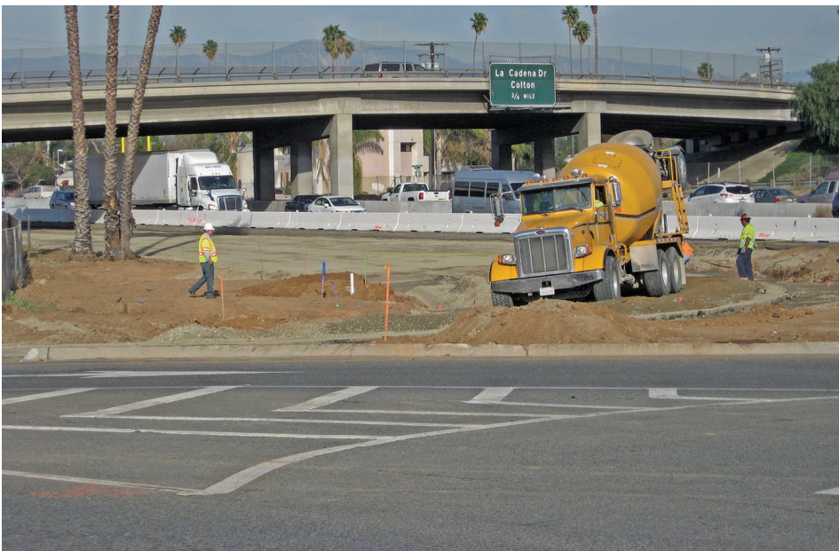
K rails blocked off the Center St. exit while new concrete was poured for the new southbound Center St. exit at Highgrove of Interstate 215.
