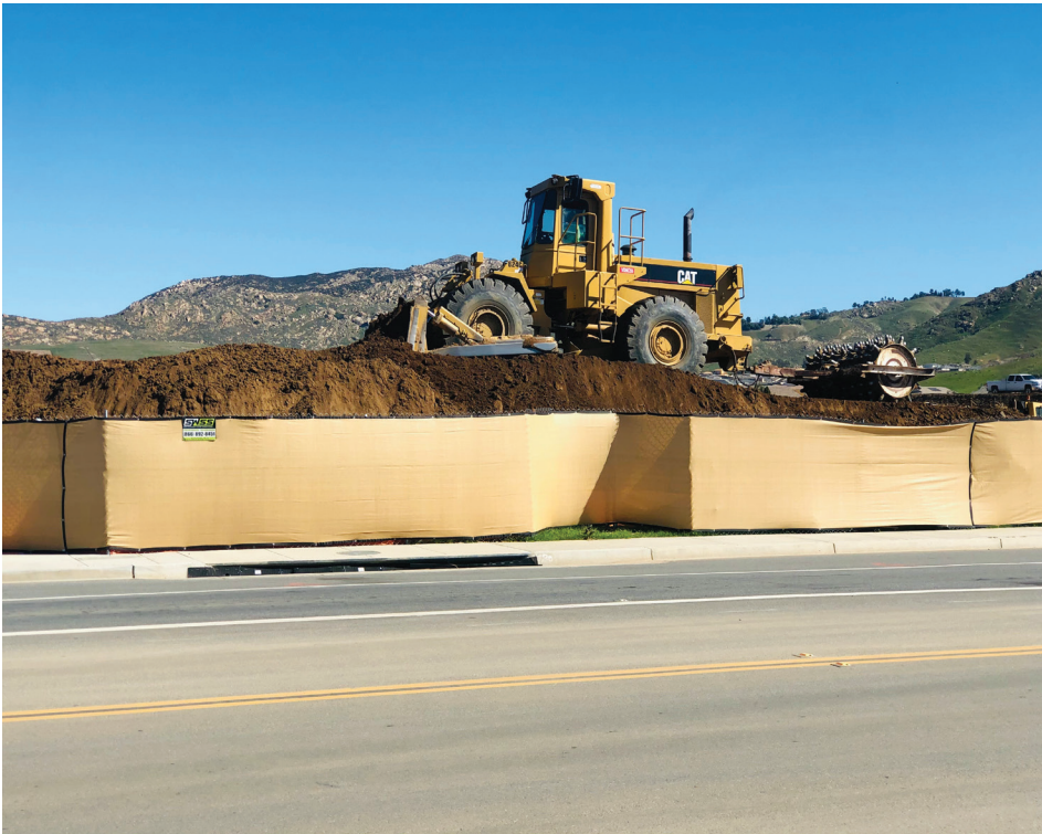
This machine is pulling a sheep's foot to compact the dirt on the south east corner of Mt. Vernon and Spring Street.
