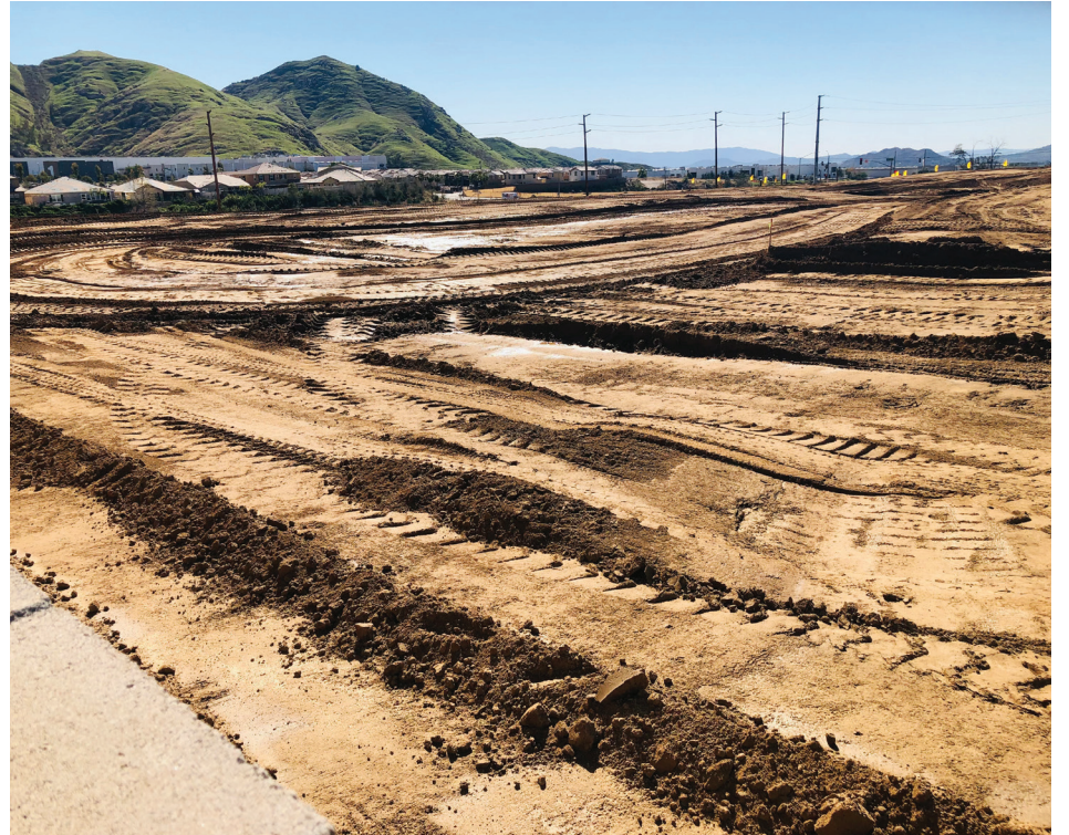
Due to the higher elevation from Mt. Vernon westward to the lower elevation by the Gage Canal, the pads for the new homes have to be terraced in order to make them level.
