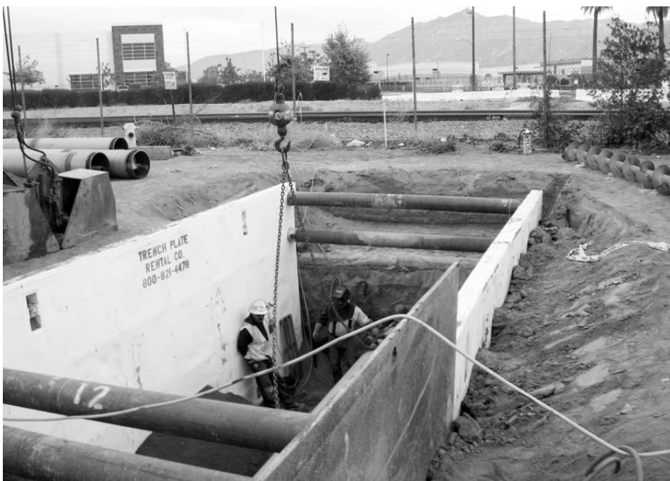
Workmen are installing a new pipe line under the BNSF Railroad main lines. This view was taken from Iowa Ave. looking eastward toward the RR tracks.
