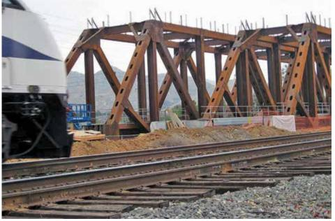
Daily Metrolink trains between San Bernardino and Riverside also use the BNSF/UP main line. The present tracks where the Metrolink train is shown will be realigned to the inside of the new steel bridges. The present bridge will be removed because it will be too short for the wider freeway.
