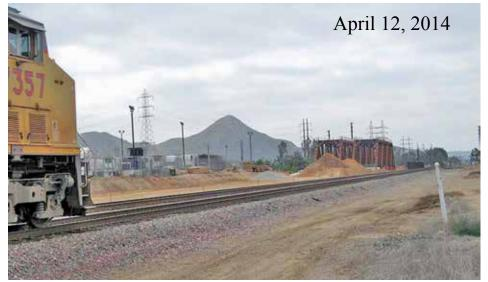
This westbound Union Pacific Freight train approaches the construction site on the existing BNSF/UP Main Line. The new Main Line will be diverted through the 2 new steel bridges when the construction and placement of the new bridges is completed.
