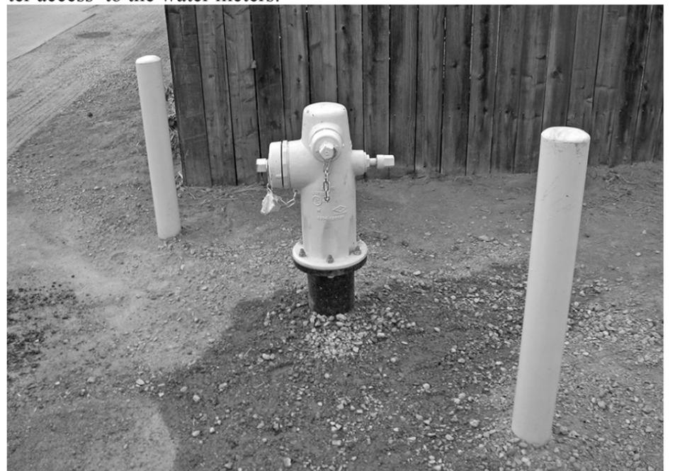
A new Fire Hydrant was also installed in this area during the water line replacement process. Villa St. has had several new homes built in this area in the last few years that was formerly known as an alleyway. Below: New safety signs are being painted in many of the streets in Highgrove.
