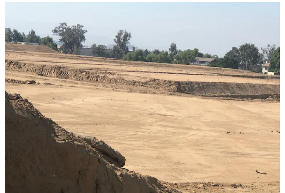
Due to the slope of the land, dirt is being moved from the east side of the properties to the west side to make the lots level..
