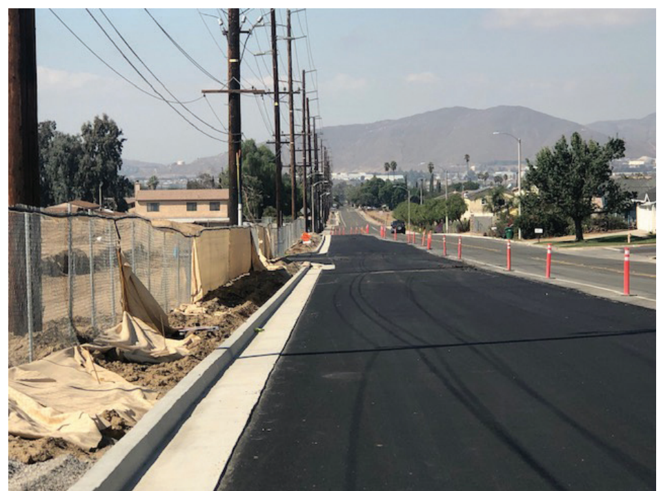
This is Spring St. looking west where the road has been widened and curbs have been added.
