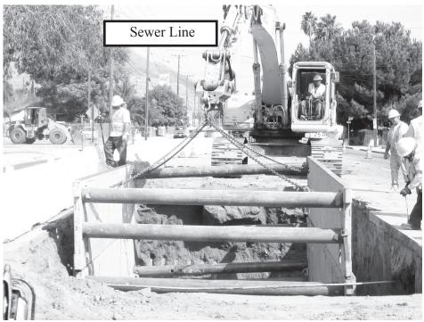
This unit is being placed in the middle of Center St. in Highgrove to prevent cave-ins when the new sewer line is drilled underneath the Riverside Canal on Center St. between Iowa Ave. and Pacific Avenue.
