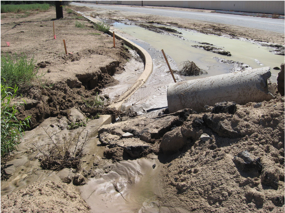
This view is looking south down Mt. Vernon Ave. where the curb is also too low for the road elevation. Rainwater and excess water from a nearby orange grove drains water into this area where it sits until it evaporates.
