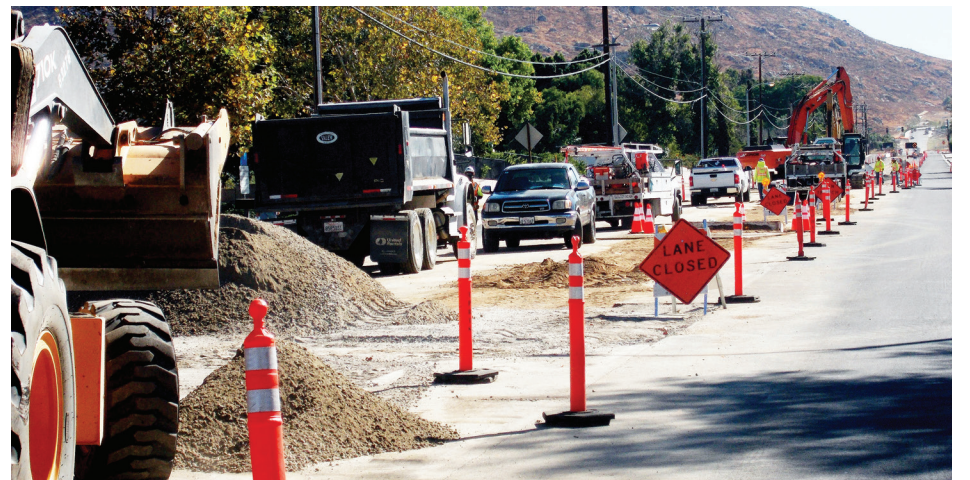
A new sewer line is being installed in the middle of Center St. from Michigan Ave. to 69 new homes at the base of Blue Mountain.
