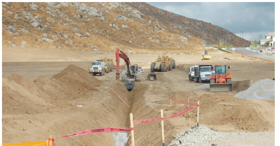
Work is being done at both ends of the sewer line. This trench is for the sewer line to connects the new homes to Riverside's sewer system.
