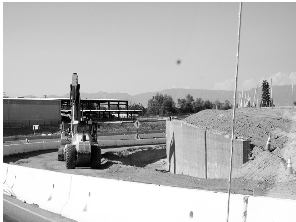
The northbound entrance to the I-215 at La Cadena Dr. is being widened and a decorative wall added on the east side. Extensive grading is underway!
